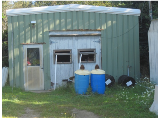
Figure 2 Matinicus Power Station
