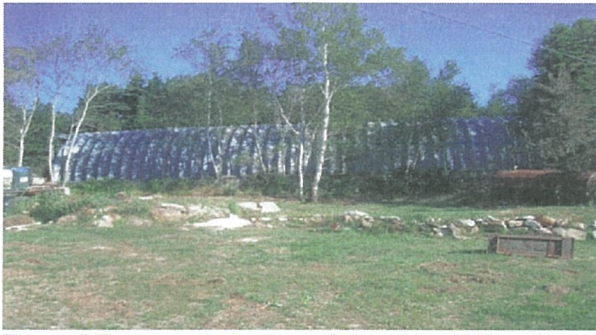
Figure 5 Town garage, proposed site of fixed PV array
