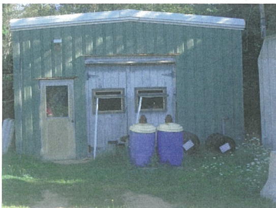
Figure 2 Matinicus Power Station
